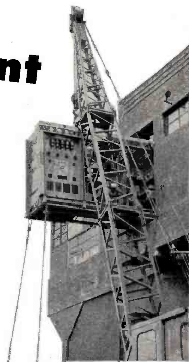
EASY DOES IT! This shot shows one of the units of the new KGW transmitter being derricked through a second story window of the transmitter house. The new installation will give KGW the most efficient transmitting equipment yet developed by the radio industry.
